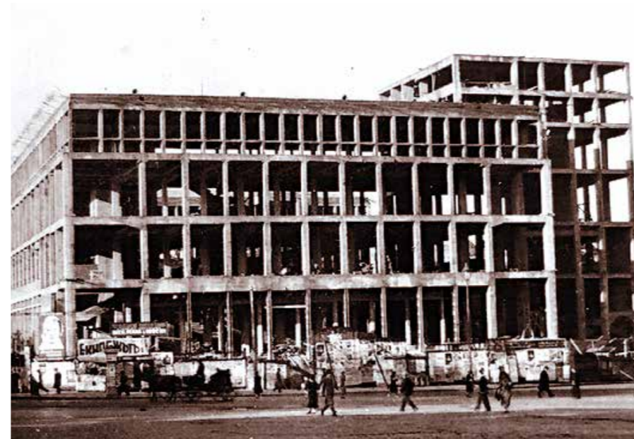
The building under construction BNB Archives
